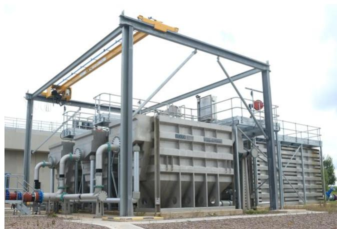
The first Mecana installation in Severn Trent to treat Nereda discharge and first in the UK with ferric dosing to a Nereda discharge to control the final effluent total Phosphorus concentration
