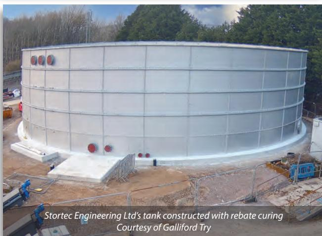
Stortec Engineering Ltd's tank constructed with rebate curing
