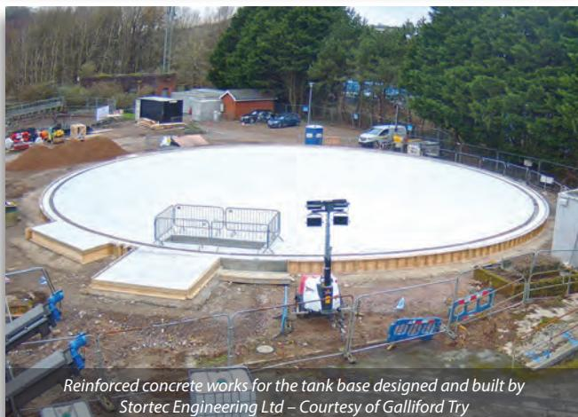
Reinforced concrete works for the tank base designed and built by Stortec Engineering Ltd - Courtesy of Galliford Try
