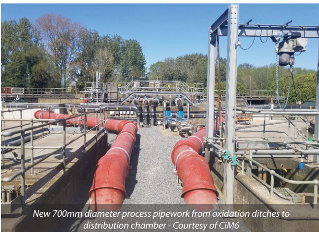
Eliquo Hydrak FBDA supplementary aerators and pipework Courtesy of CiM6
