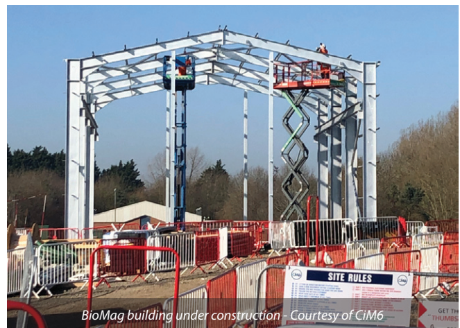
BioMag building under construction - Courtesy of CiM6
