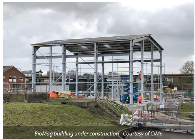
BioMag building under construction - Courtesy of CiM6
