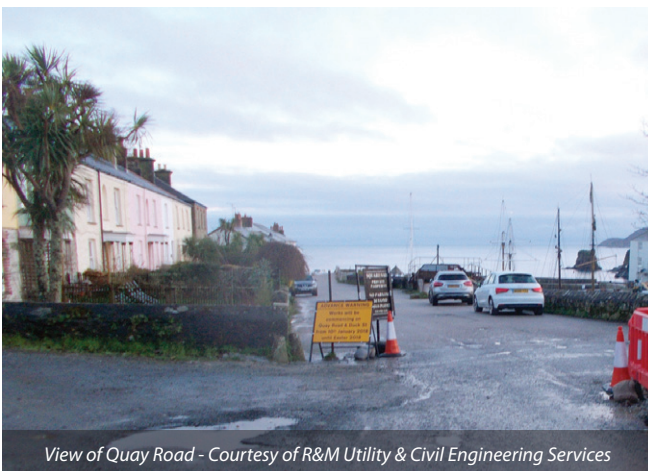
Pipex pumping station manhole chamber Courtesy of R&M Utility & Civil Engineering Services
