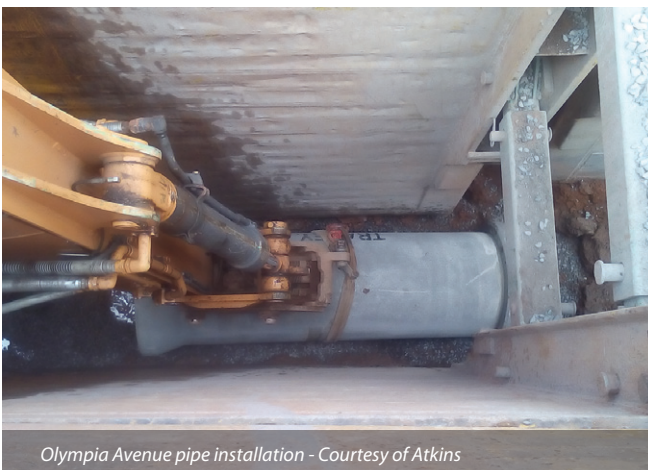
Olympia Avenue open cut works - Courtesy of Atkins
