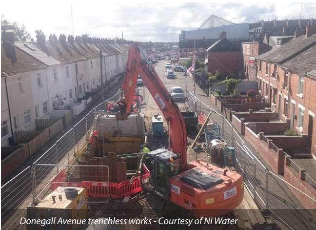
Donegall Avenue auger boring - Courtesy of Atkins
