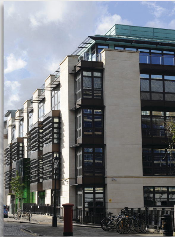
Image 2: Horizon House: The Environment Agency's Head Office in Bristol utilises rainwater harvesting and recycling to flush water efficient toilets, reducing total mains water use by 70% - Courtesy of AECOM
