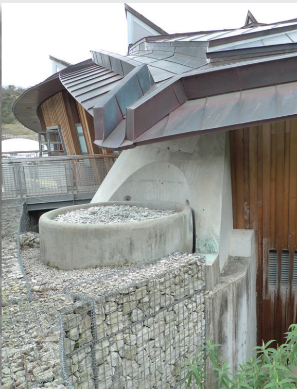
Image 3: Rainwater collection at the Eden Project's 'Core' building, Cornwall. Water sensitive measures adopted across the site include rainwater harvesting for toilet flushing and irrigation, surface water infiltration, water efficient fittings and water cycle education Courtesy of AECOM
